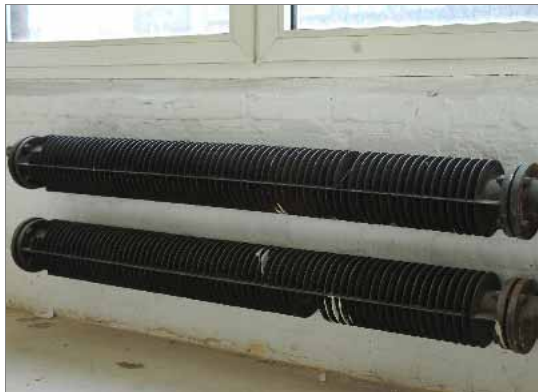
Original Röhren-Radiator
